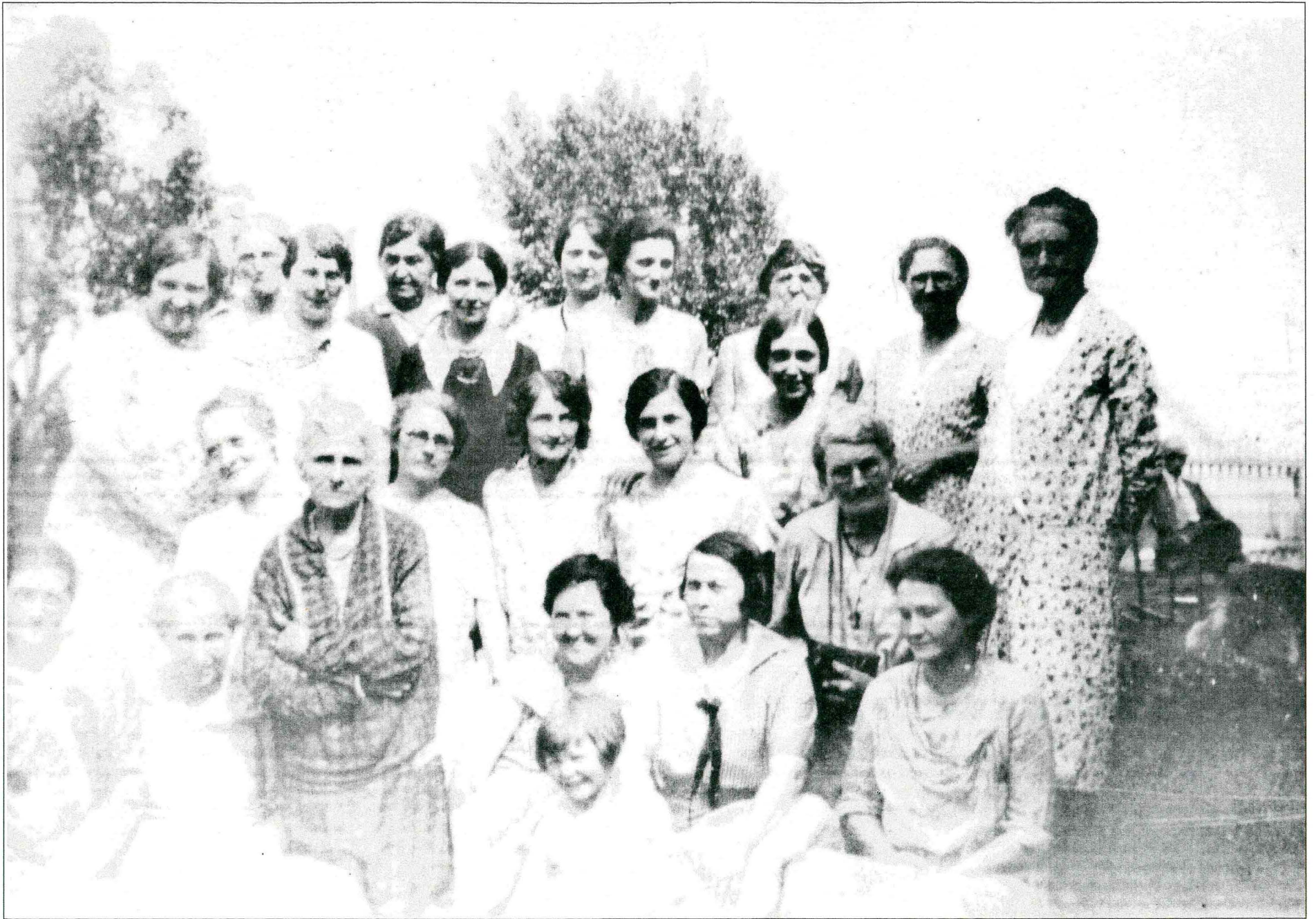
Frankfort Springs United Presbyterian, Frankfort Presbyterian and King's Creek United Presbyterian
