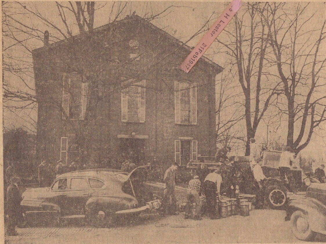
Historic Cross Creek Presbyterian Church, at Cross Creek, was damaged by fire yesterday. Flames destroyed the bell tower atop the edifice and damaged the roof. District fire departments and volunteers rushed to the scene, being shown in front of the church yesterday in the picture above.
